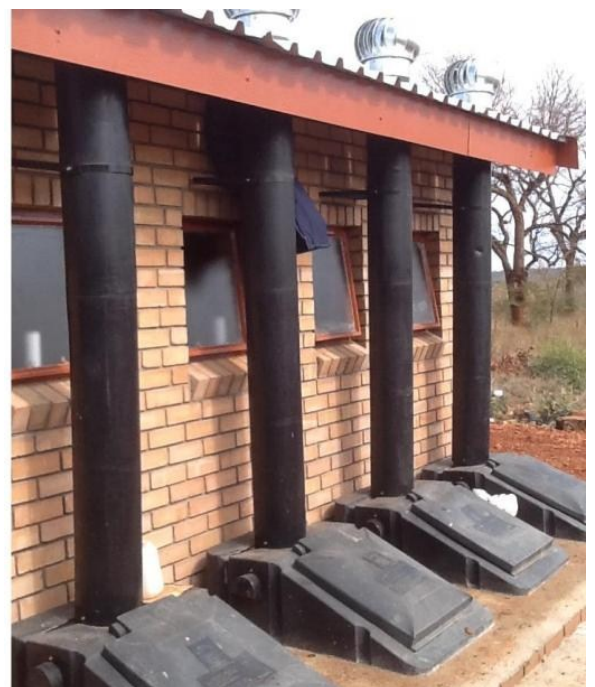
Biogas Toilets in Ghana
